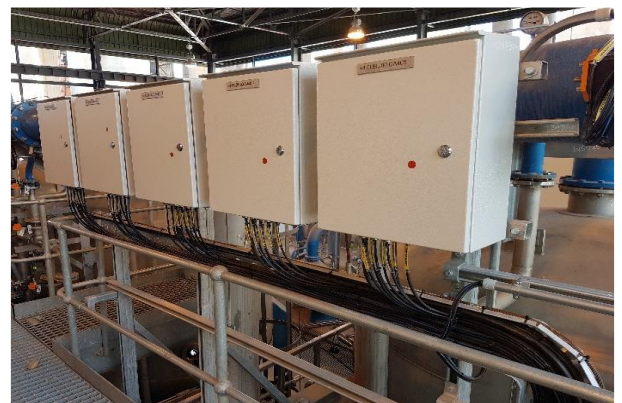
Installation of JB's, Racking and Cabling
