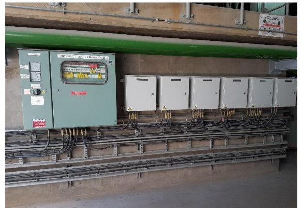
Installation of DB's ,Racking and Cabling
